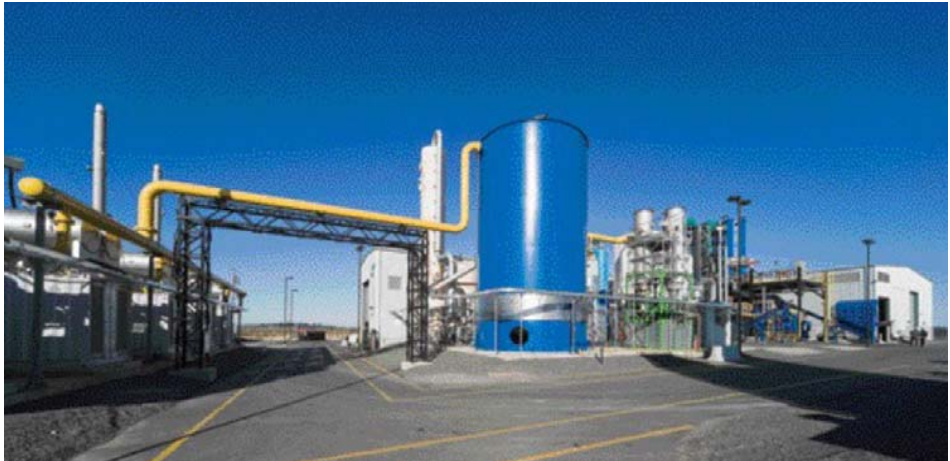
Plasco Conversion System - Ottawa, Canada
