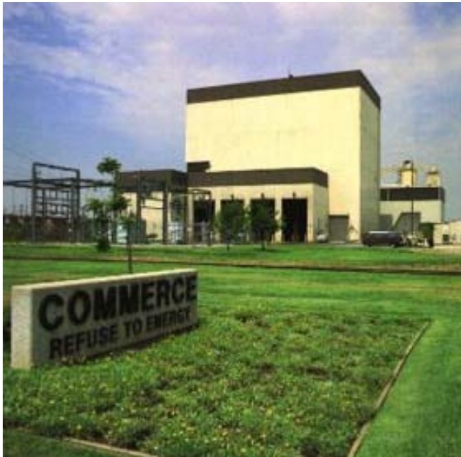
Refuse to Energy Facility, City of Commerce
